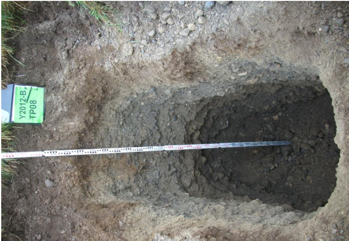
Trial Pit Side/Base
