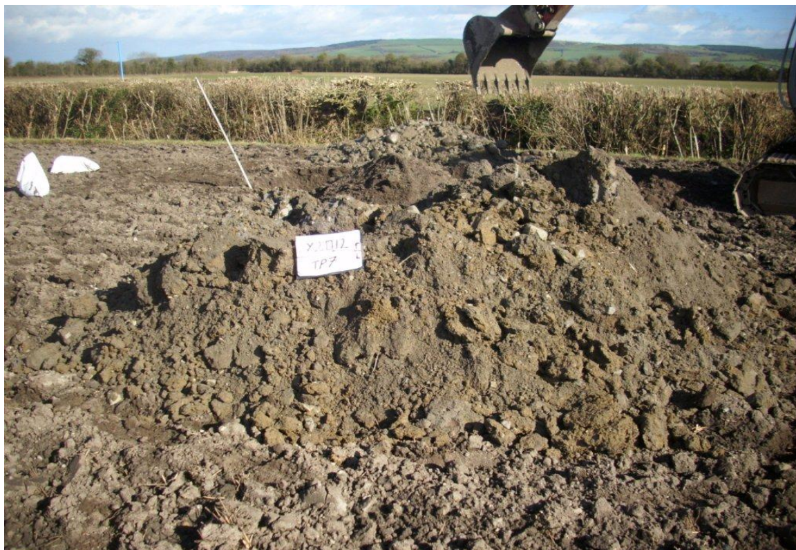
Trial Pit Spoil
