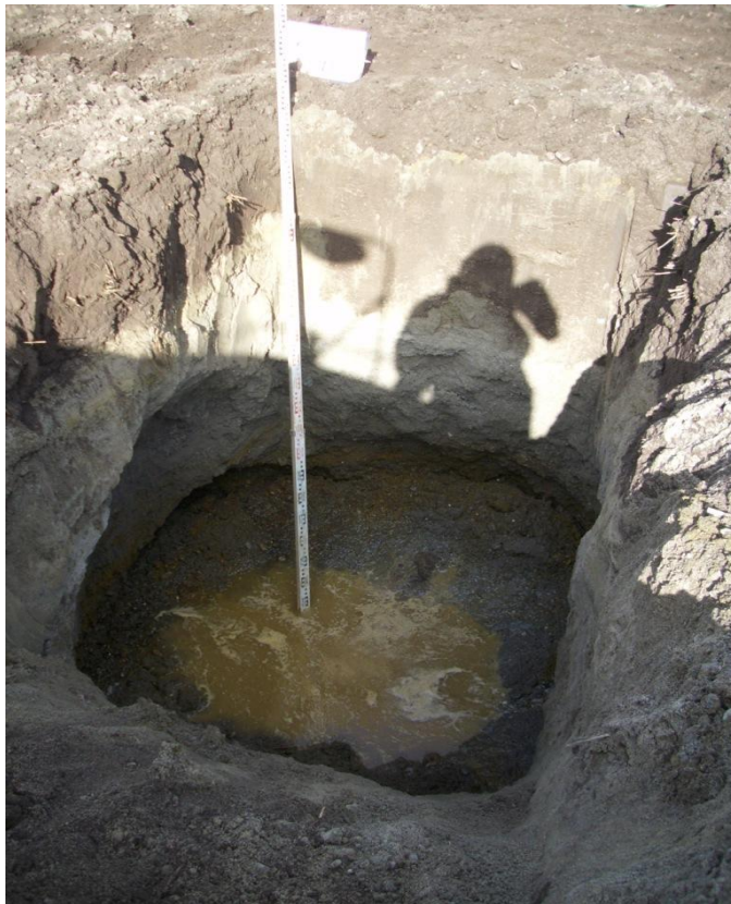
Trial Pit Side/Base
