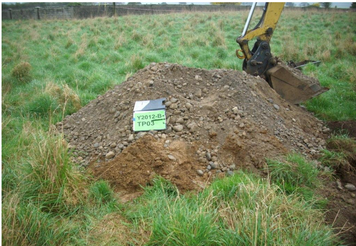
Trial Pit Spoil
