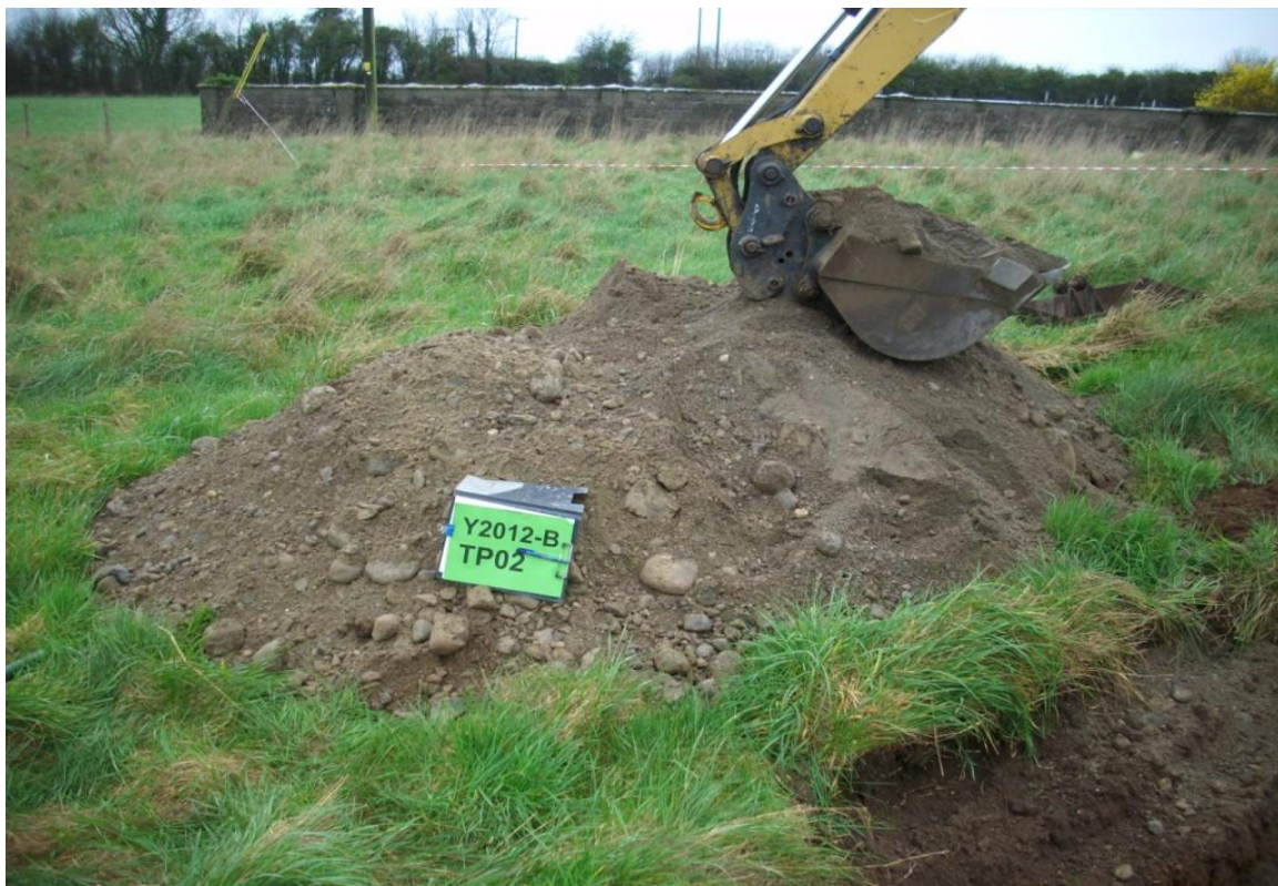
Trial Pit Spoil
