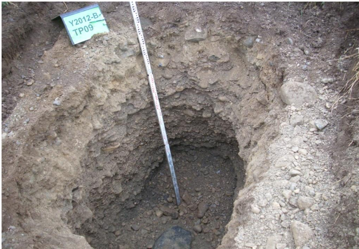
Trial Pit Side/Base
