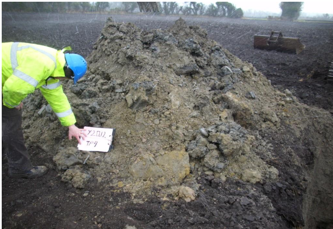
Trial Pit Spoil
