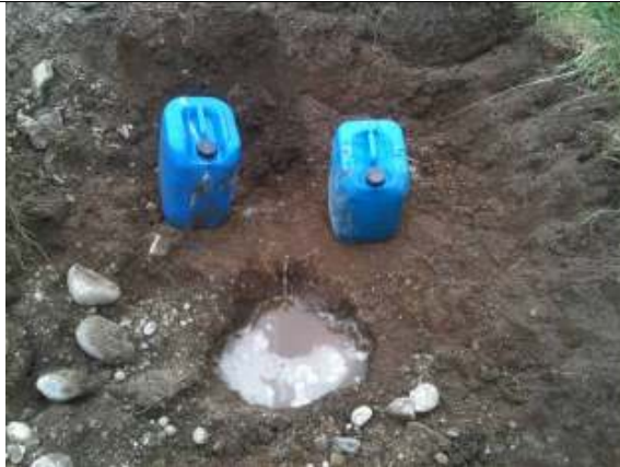
Percolation ("T") Test 3
