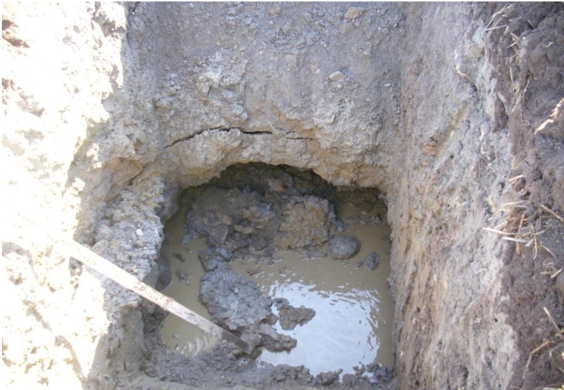
Trial Pit Side/Base
