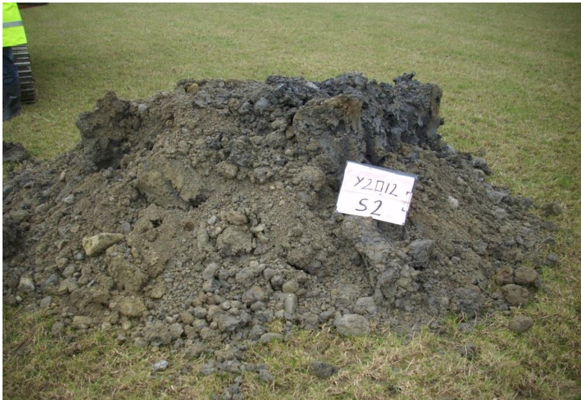
Trial Pit Spoil
