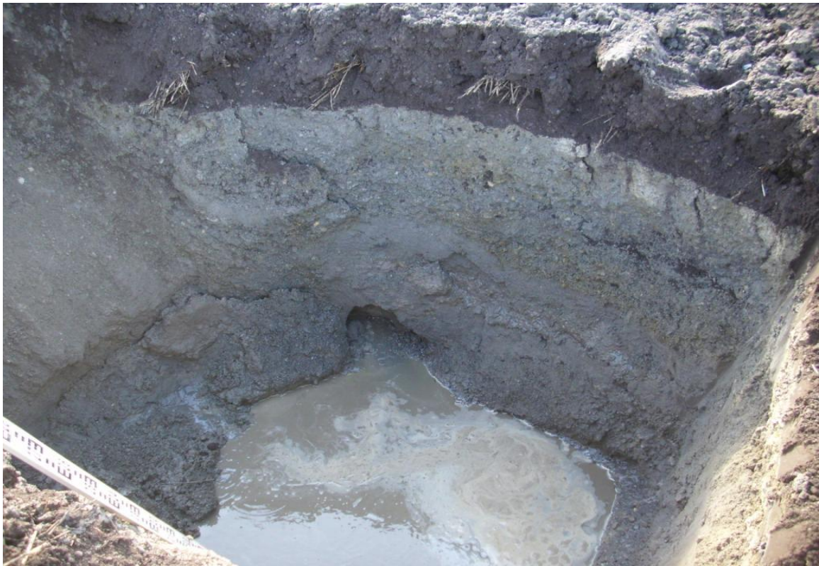
Trial Pit Side/Base
